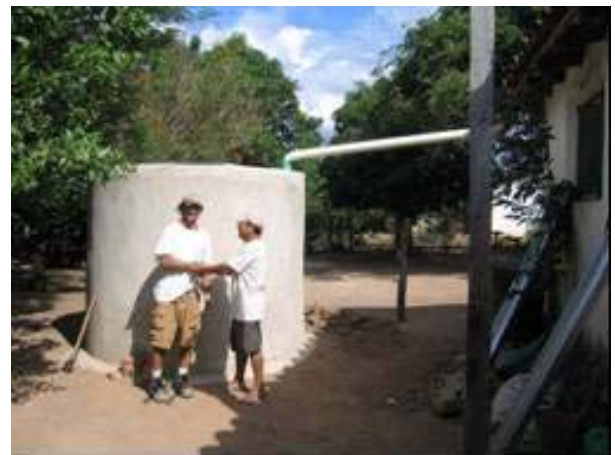
Rainwater catchment system constructed by PCV Stephen Lotti .
